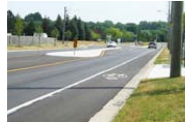
Bike lane on Davenport Rd
