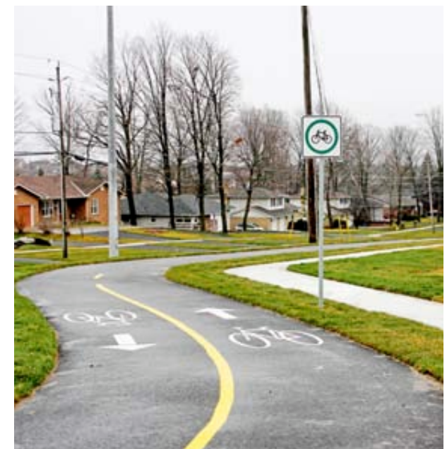
The two-way bike trail and sidewalk on the west side of the street is separated to avoid conflicts between pedestrians and cyclists.
