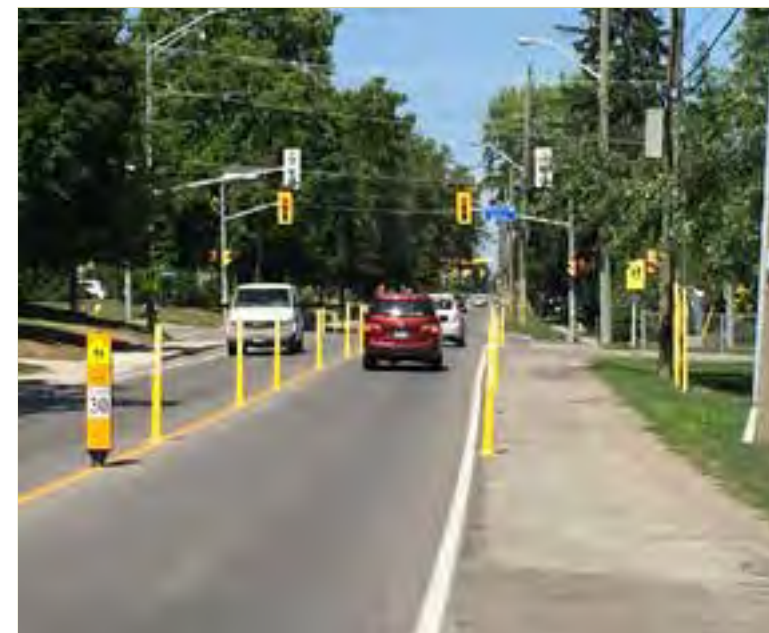
Traffic calming using flexible bollards in Pelham, ON.
